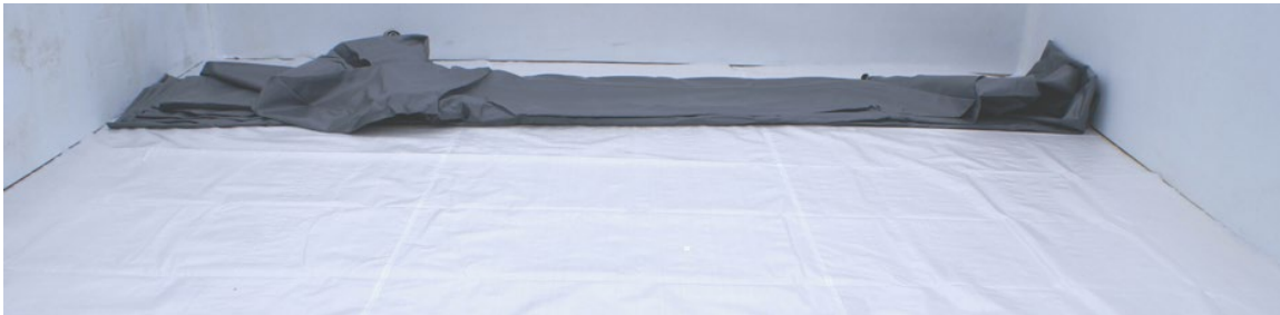
Figure 32 – Unfolding the liner
