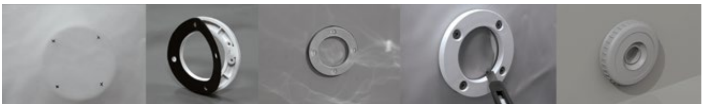
Figure 34 – Installing the return fitting flange
