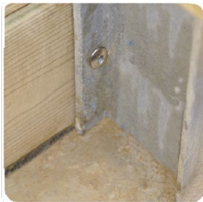
Figure 9 – Fastening the slats to the supporting braces
