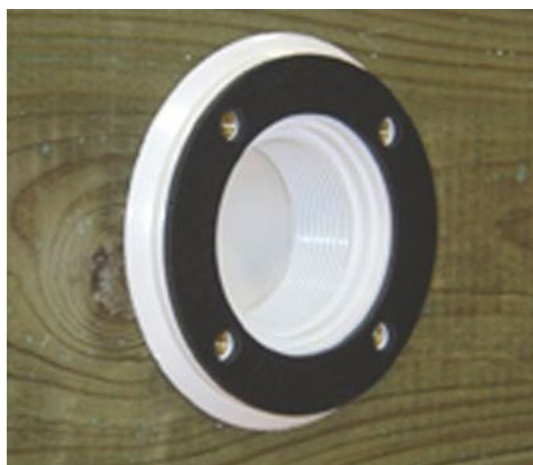
Figure 24 – Mounting the return fitting body and gasket
