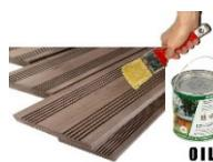
To protect wood from weather, it is advisable to apply preparations intended for the protection of external wooden constructions (e.g. oil scumble which is available in the current offer - product developed for the effective protection of wooden swimming pools). Pool preservation should be performed at least once a year, and for pools subject to extreme weather conditions even more often.
