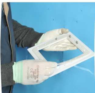
Place the seal over the flange
