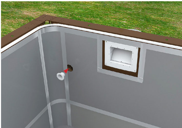
The outlet nozzle is placed in the hole conceived for this purpose.
